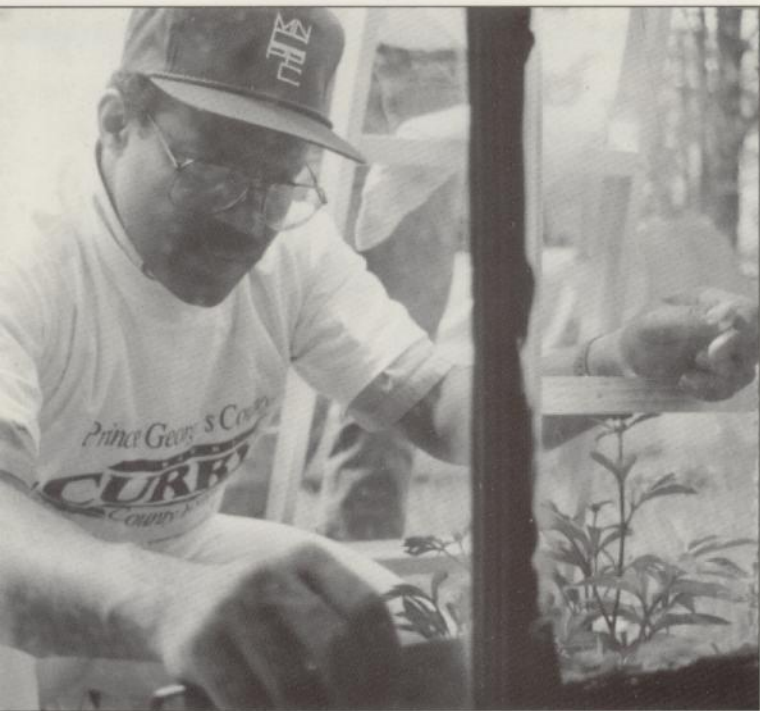
Wayne Curry repairs window on senior citizen's home in College Park.
