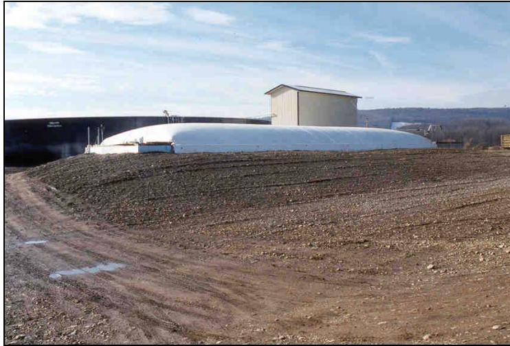
Figure 4. Plug Flow AD System
